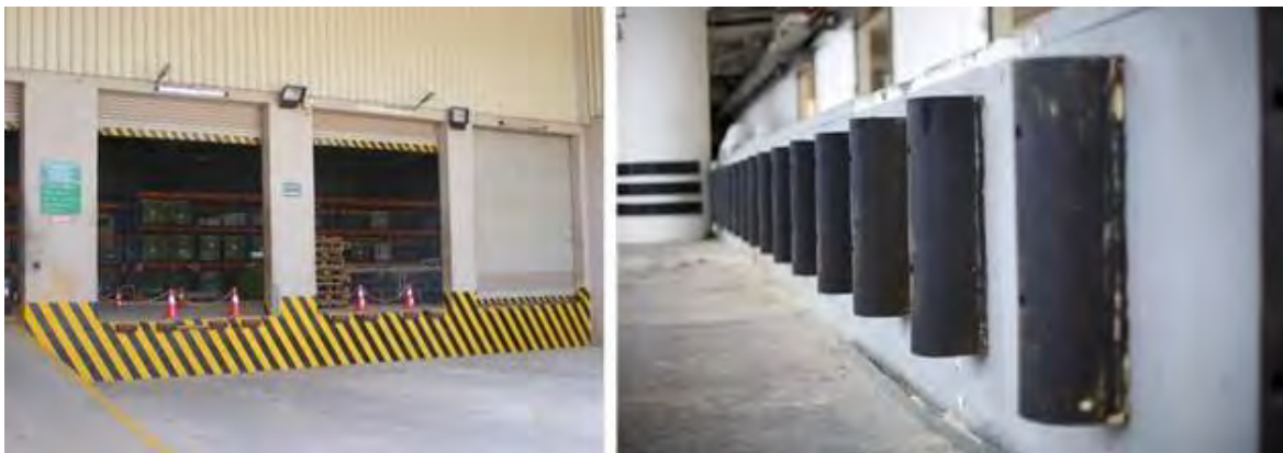
Fig 1.5.7: Loading/ Unloading bay
